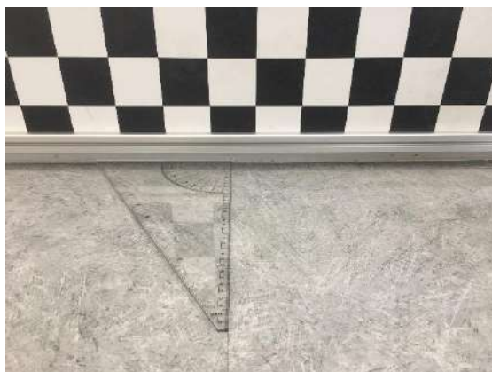
Finding a line perpendicular to the wall
